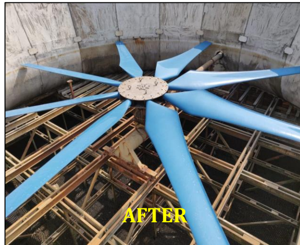
Replacement of CT Fan blades with redesigned blades
