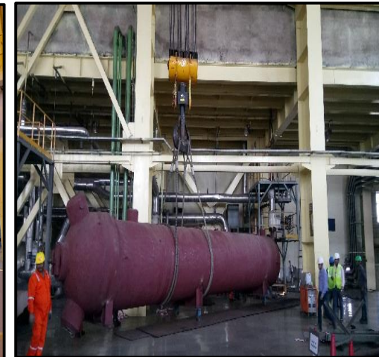
Installation of HPH-6 after refurbishment of tube bundle
