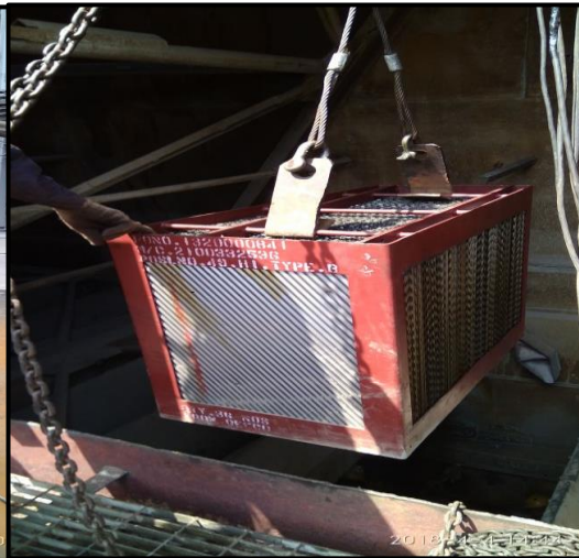
Installation of new basket
