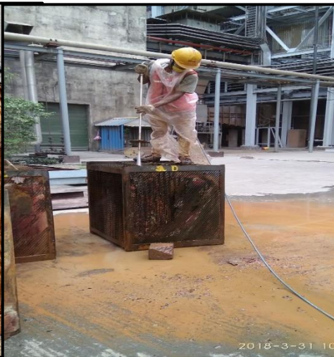
High pressure water jet cleaning of basket
