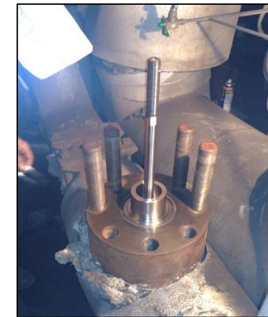
Upgradation of BFP RC valve trim set from single stage to multistage
