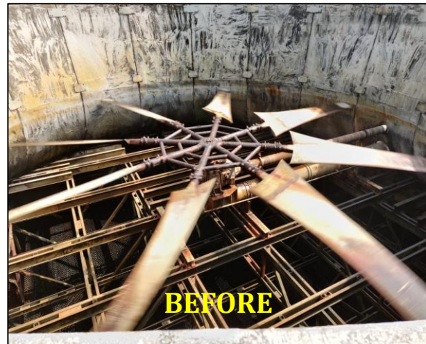
Replacement of CT Fan blades with redesigned blades
